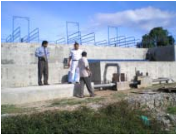
Photo 5 ETP Ashroff Memorial Hospital
