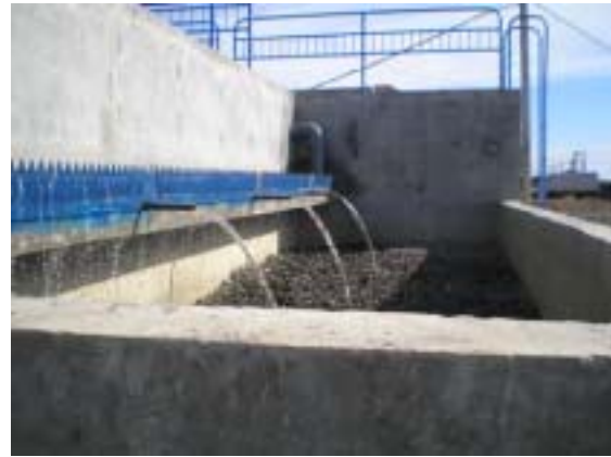
Photo 6 Effluent ETP Ashroff Memorial Hospital
