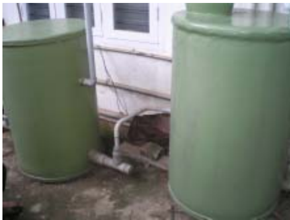
Photo 6 PAB reactor in India
