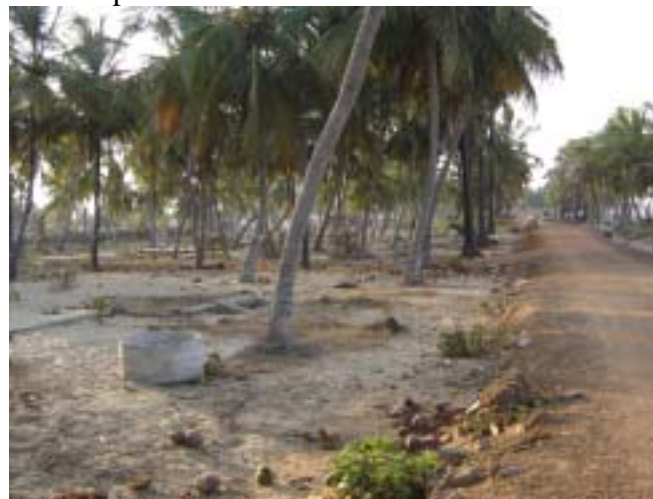
Photo 5 Road constructed by using debris in Kalmunai (Energy Forum)
